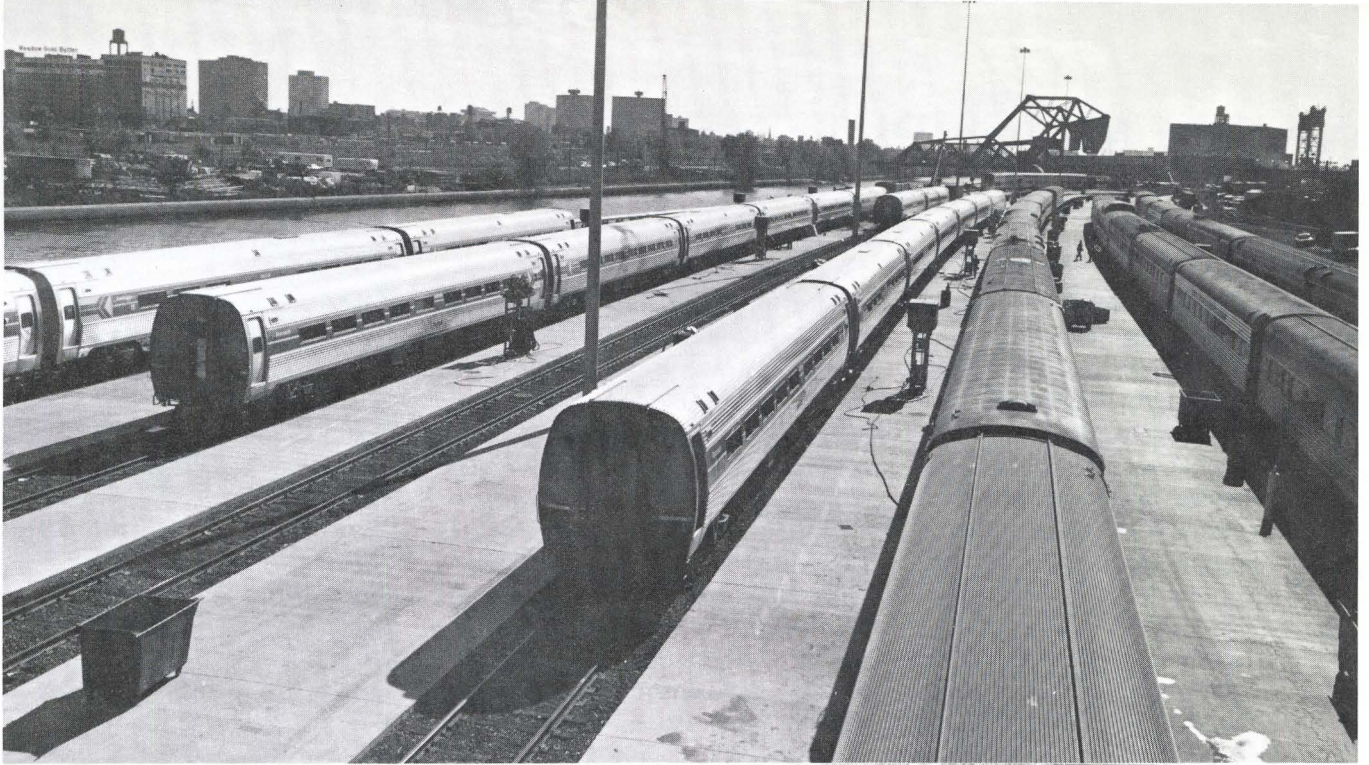
A portion of the new coach yard, stretching south of Roosevelt Road and consisting of seven tracks, has been completed and put into use.
