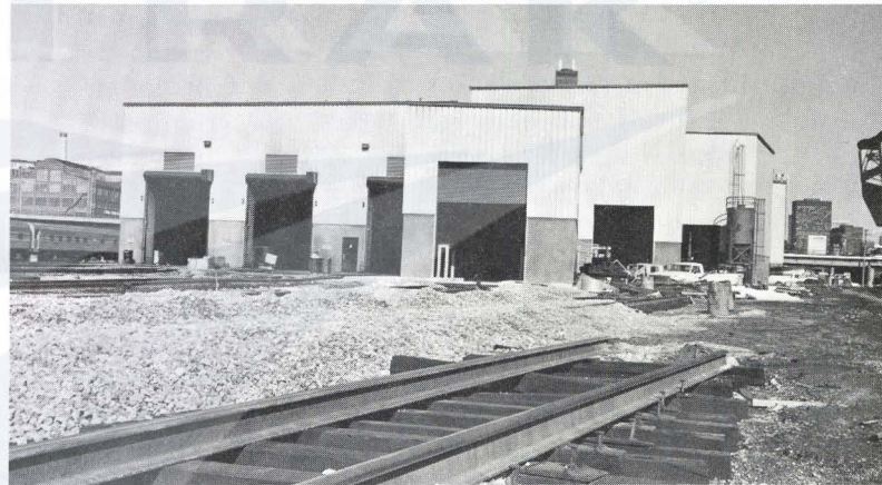
The new diesel repair building will do most of the heavy repair work on Amtrak's diesel fleet.
