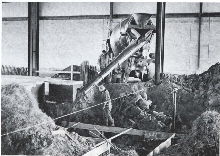
Cement is poured inside facility for track bed.
